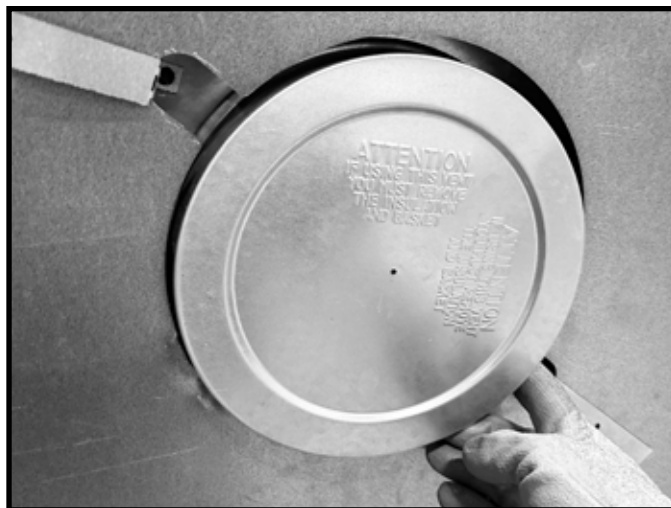
Figure 6.14 Fold the straps away from cap. Remove seal cap utilizing cutouts.
