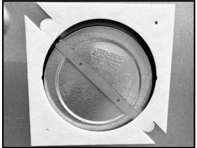
Figure 6.12 Remove the insulation gasket by bending tabs in and pulling gasket piece out.
