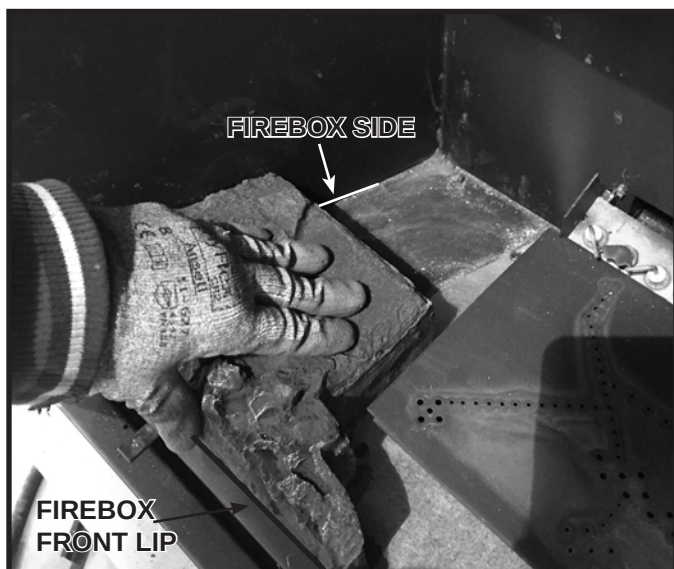
Figure 11.2 Install Left Hearth Component
