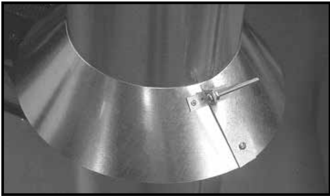
Figure 7.13 Insert Bolt into Brackets
