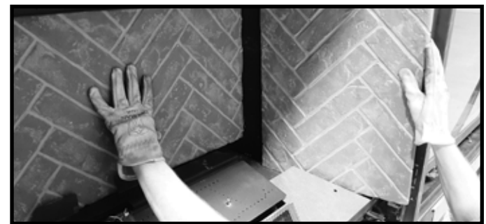
Figure 11.3 Install Side Refractory Panel (Right Side Shown)
