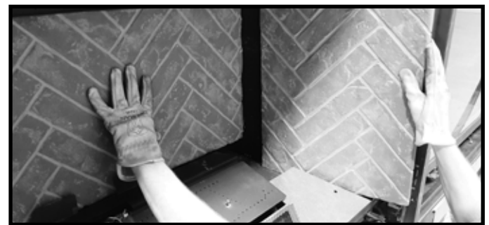
Figure 11.3 Install Side Refractory Panel (Right Side Shown)
