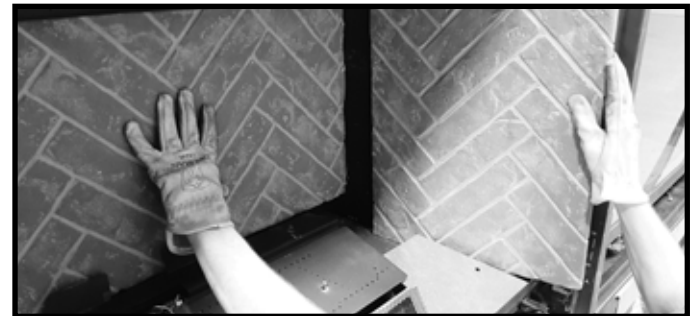
Figure 11.3 Install Side Refractory Panel (Right Side Shown)
