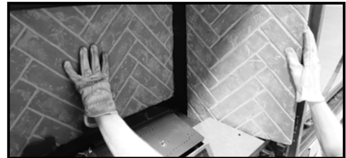
Figure 11.3 Install Side Refractory Panel (Right Side Shown)
