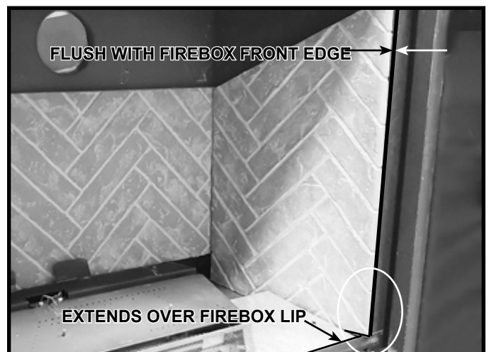
Figure 11.4 Side Refractory Panel Installed (Right Side Shown)
