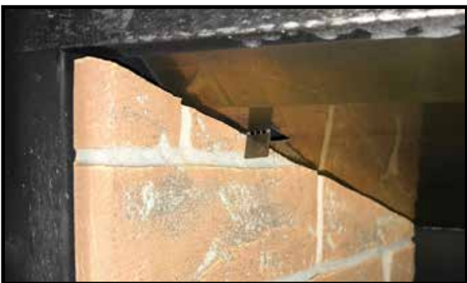
Figure 6 Left Refractory Handbend Tab
