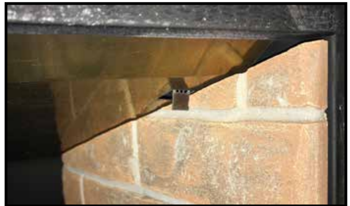
Figure 7 Right Refractory Handbend Tab
