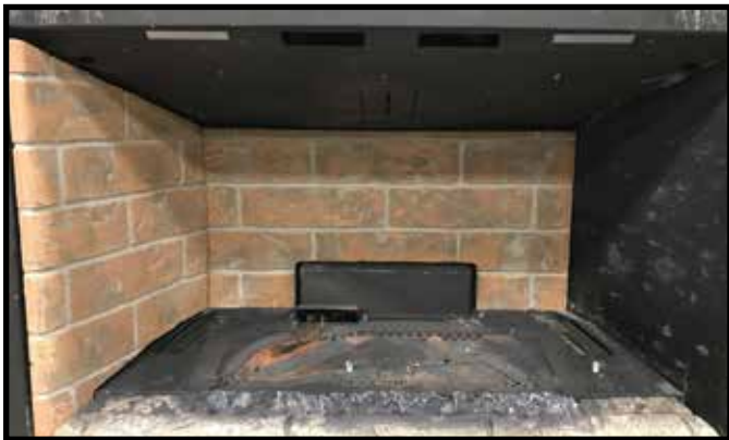
Figure 5 Left Refractory Installed
