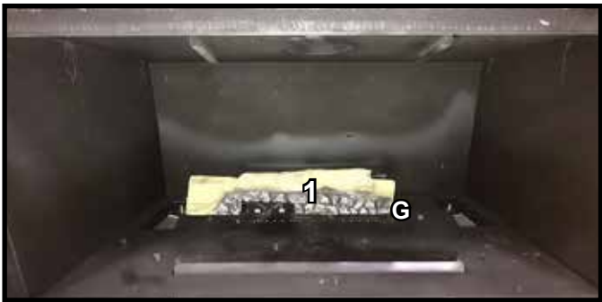
Figure 3. Log #1 Installed
