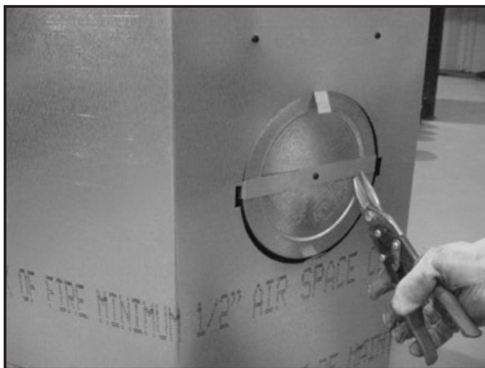
Figure 6.7 (Generic Fireplace Shown) Cut the metal retaining band and fold the sides out.
