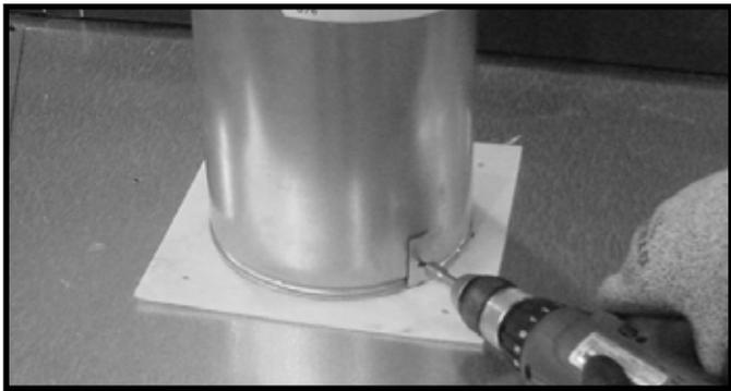
**Figure 6.6 (Generic Fireplace Shown)** To attach the first section of vent pipe, make sure to use the fiberglass gasket in the manual bag to seal between the first vent component and the outer fireplace wrap. Use 2 self tapping screws to secure the gasket to the outer wrap.
