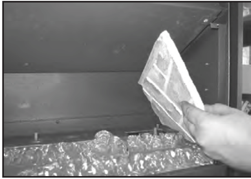
Figure 8.4 Install left and right brick panels. Place in lower channels and push toward the side.
