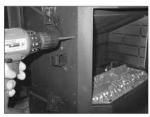
Figure 8.3 To remove existing metal refractory remove the two screws located on the left and the two on the right sides behind the side curtains.
