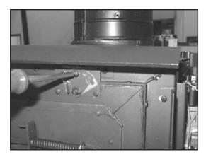
Figure 8.13 The vertical damper adjustment is located on the right side of the unit behind the side curtain. The damper is centered towards the top of the unit.
