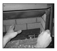
**Figure 8.6** Install the left and right brick panels. Use the screw placement shown in **Figure 8.3** to secure them in place. Reassemble appliance.
