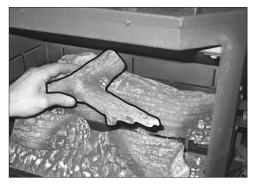
Figure 8.10 Place twig over the locator pin on the rear log, gently laying the log across the two front logs. To complete your log set application reinstall the front of the unit.
