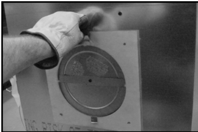
Figure 6.7 (Generic Fireplace Shown) Fold the tabs toward the center of the seal cap (90°) and remove the insulation gasket.
