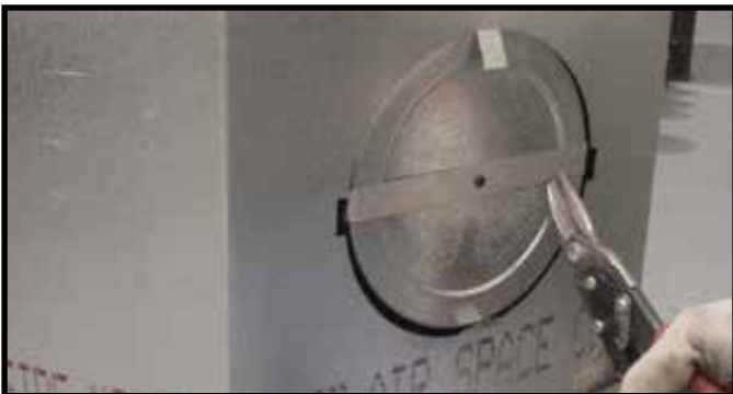
Figure 6.9 Cut the metal retaining band and fold the sides out.
