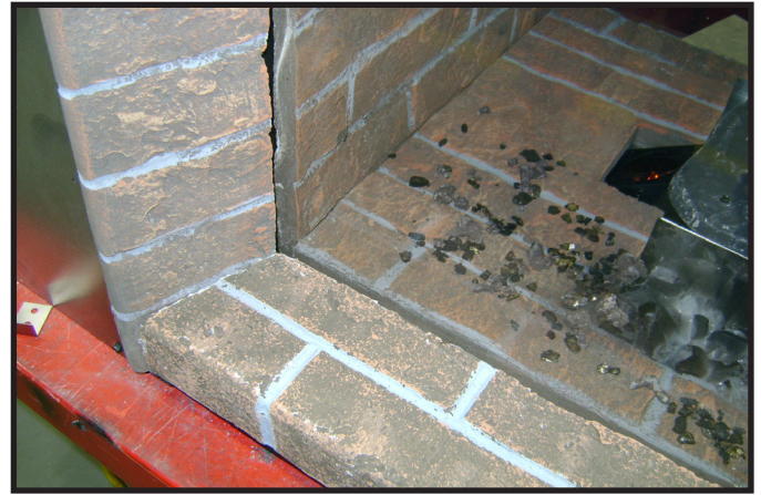
Figure 11.28 Outer Hearth Installation
