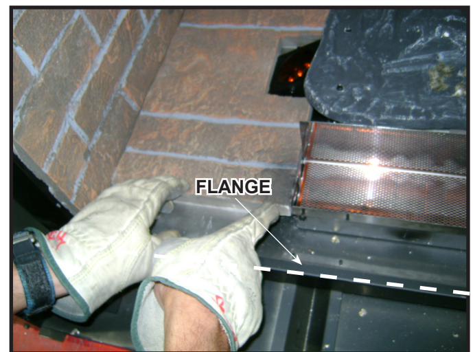
Figure 11.18 Positioning Left and Right Middle Base Refractory
