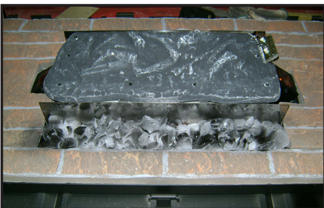
Figure 11.22 Finished Ember Bed
