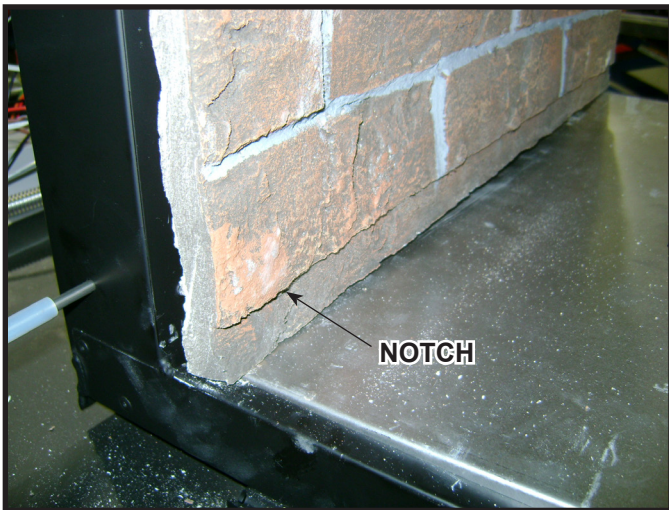
Figure 11.15 Notched End of Side Refractory
