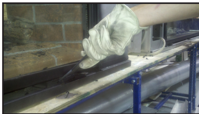
Figure 11.3. Inserting Glass Clip Tool
