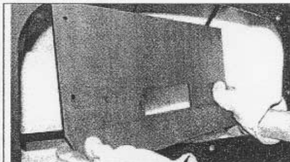
Figure 9A Placing Restrictor Plate
