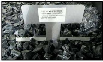
Figure 9.7 Rock Placement Jig
