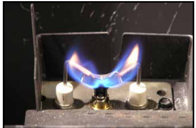
Figure 3.1 IPI Pilot Flame Pattern
