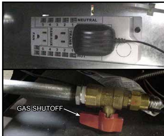
Figure 13.1 Red Gas Shutoff Knob
