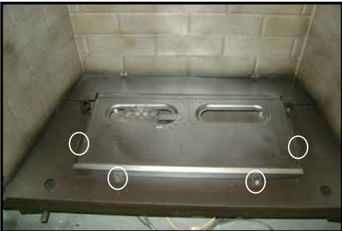
Figure 3.9 Remove Burner Skirt
