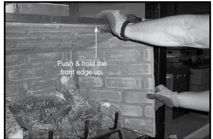
Figure 7.9 Remove One Side Refractory
