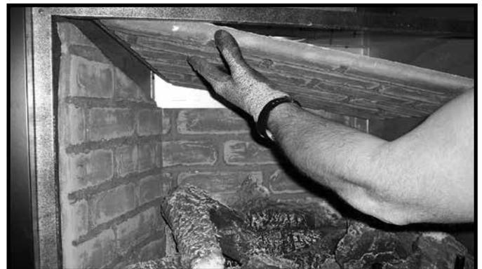
Figure 7.10 Remove Top Refractory
