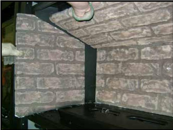
Figure 3.2 Top Refractory Removal
