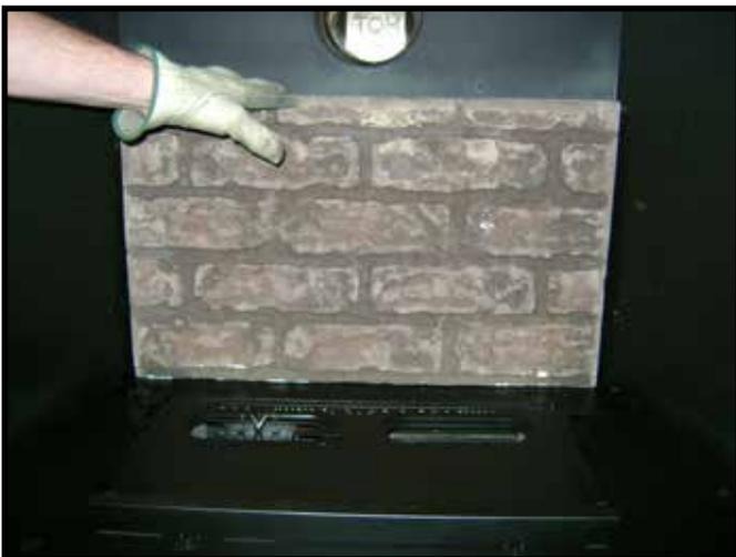
Figure 3.4 Back Refractory Removal
