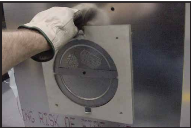
Figure 6.8 Fold the tabs toward the center of the fire plug (90°) and remove the insulation gasket.
