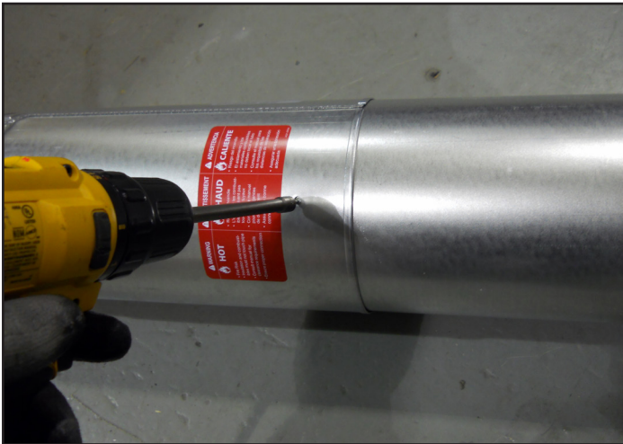
Figure 7.4 - Screws into Slip Section
