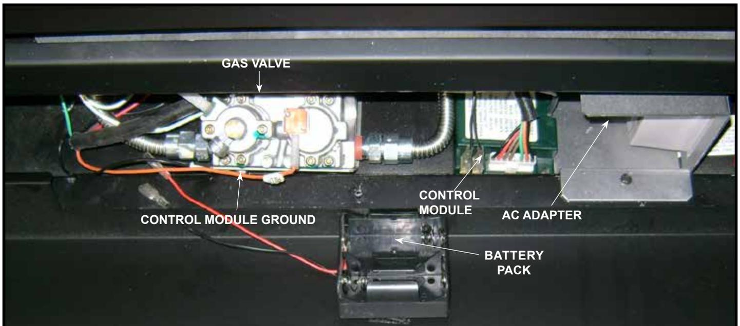
Figure 12.1 Valve Cavity
