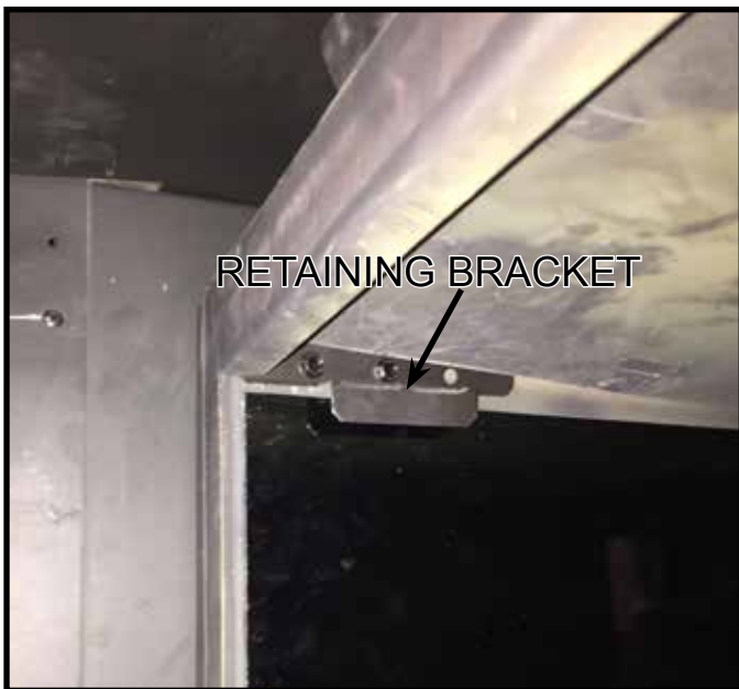
Figure 5 Retaining Bracket Installation - Side Panel
