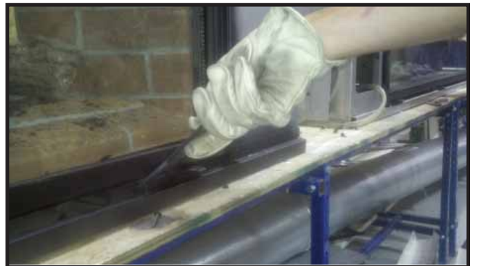
Figure 14.3 Inserting Glass Clip Tool
