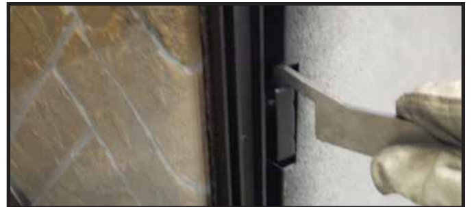
Figure 14.7. Fasten Side Glass Clips
