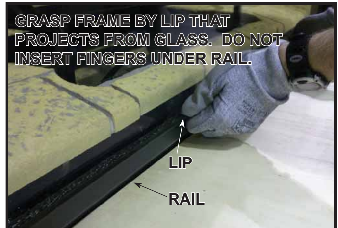
Figure 14.6. Install Glass
