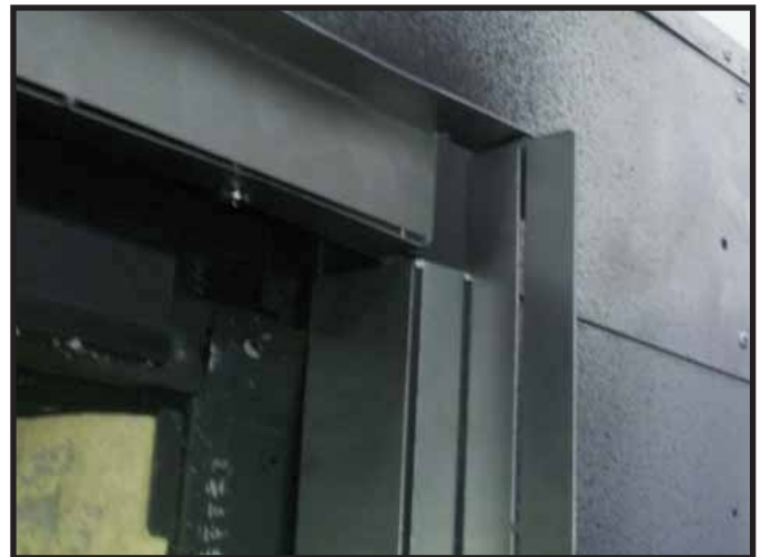
Figure 13.4 Top/Side Finishing Templates Installed
