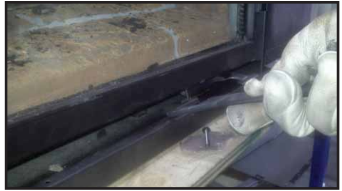
Figure 14.2 Glass Clip Tool Location
