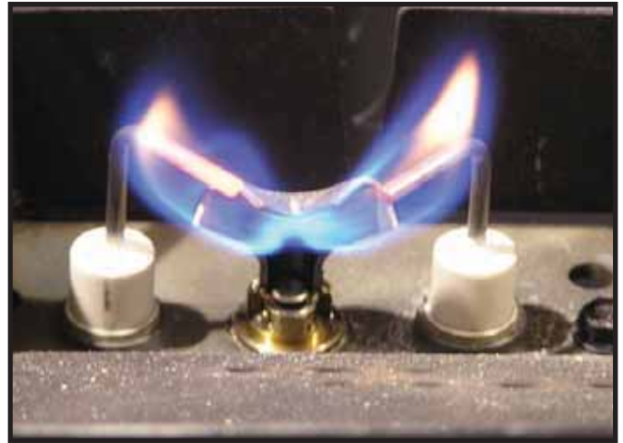
Figure 3.1 IPI Pilot Flame Patterns
