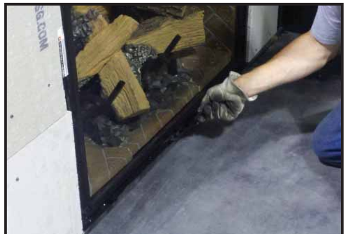
Figure 14.8. Fasten Lower Glass Clips
