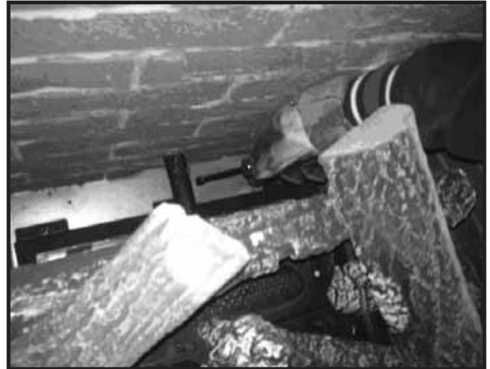
Figure 1. Air Shutter Location
