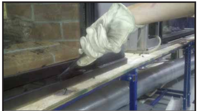
Figure 14.8. Inserting Glass Clip Tool
