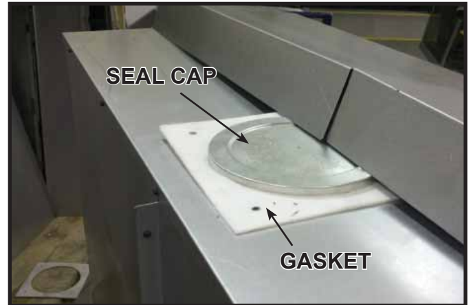
Figure 9.2 Seal Cap and Gasket Location
