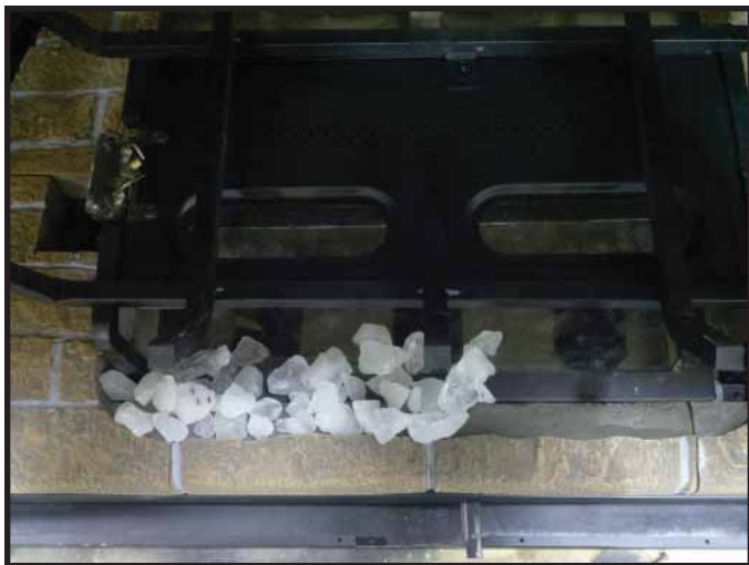
Figure 14.1. Install Teco-Sil
