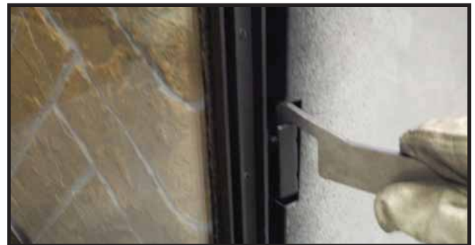
Figure 14.12. Securing Side Glass Clips
