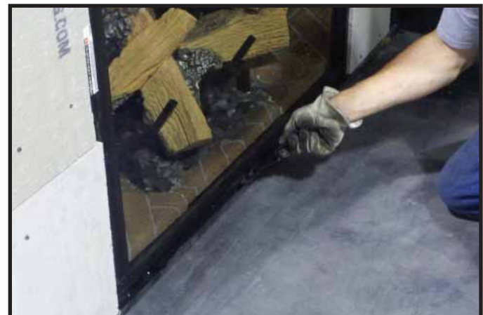
Figure 14.13. Securing Bottom Glass Clips
