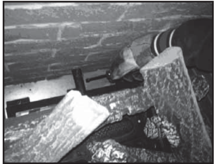
Figure 1. Air Shutter Location
