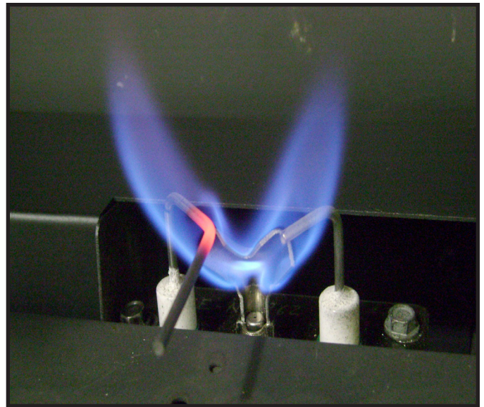
Figure 3.1 IPI Pilot Flame Patterns
