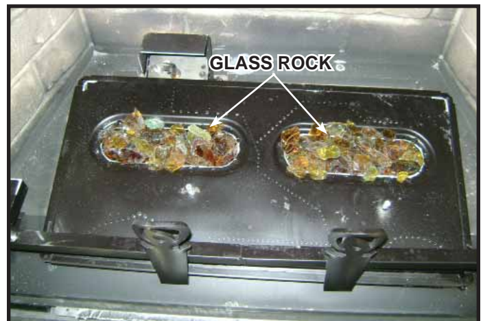
Figure 3. Install Glass Rock
