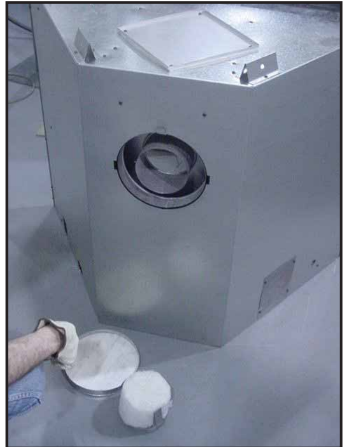
Figure 9.10 Discard the vent cap, remove and discard the insulation basket.
