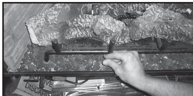
Figure 14.4 Placement of Vermiculite
