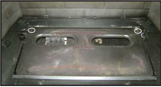
Figure 3.8 Remove Screws from Burner Assembly Rear Corners
