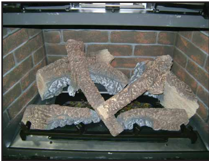
Figure 1. Log Set Installed
