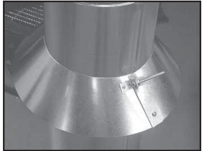
Figure 8.7 Assembling the Storm Collar Around the Pipe
