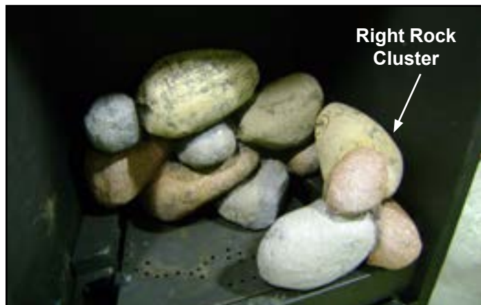
Figure 8.16 - Placing Right Rock Cluster
