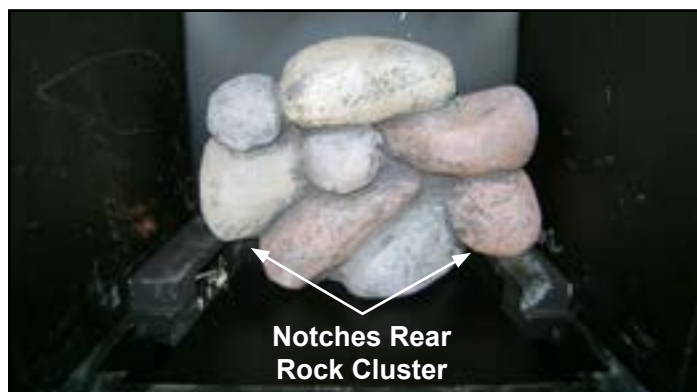
Figure 8.15 - Placing Rear Rock Cluster
