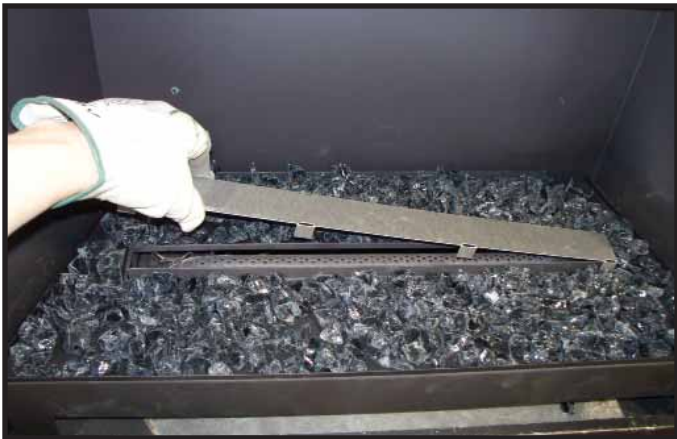
Figure 5. Removing Rock Media Jig.
