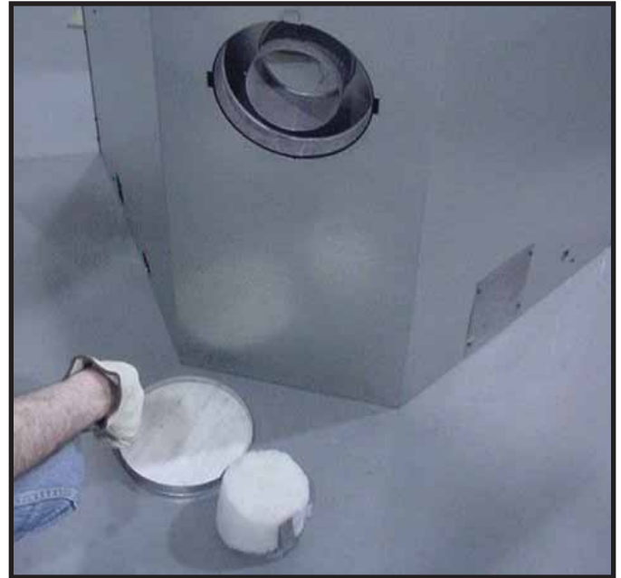
Figure 9.10 Discard the vent cap, remove and discard the insulation basket.
