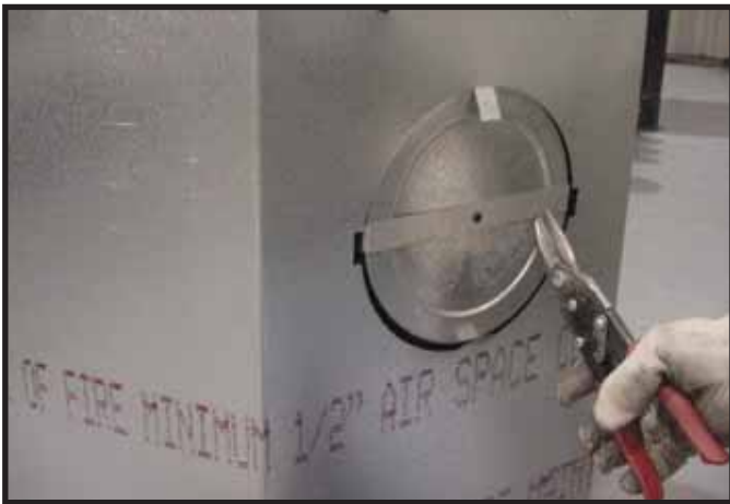
Figure 9.8 Cut the metal retaining band and fold the sides out.
