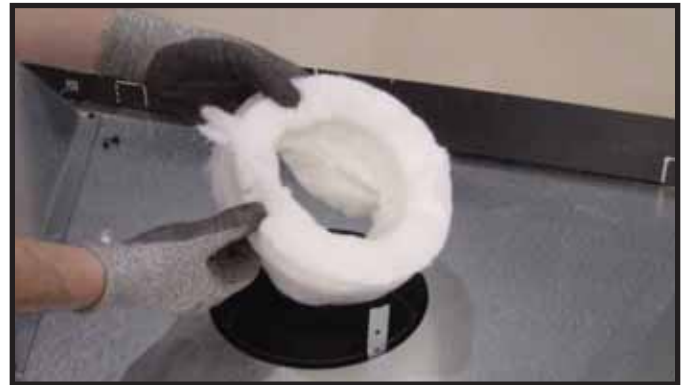
Figure 9.5 Remove the insulation from the outer vent pipe. For rear venting there is no insulation in the outer vent pipe.
