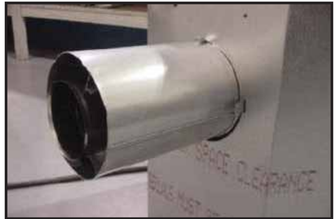
Figure 9.11 Attach the first vent section (it will snap into place). Slide the insulation gasket onto the vent section, up against the appliance and over the tabs.
