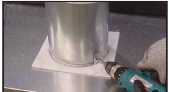
Figure 9.6 To attach the first section of vent pipe, make sure to use the fiberglass gasket in the manual bag to seal between the first vent component and the outer fireplace wrap. Use 2 self tapping screws to secure the gasket to the outer wrap.
