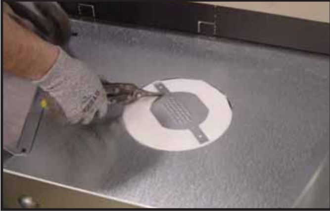
Figure 9.1 Cut the seal cap strap across the rectangles next to the disk.
