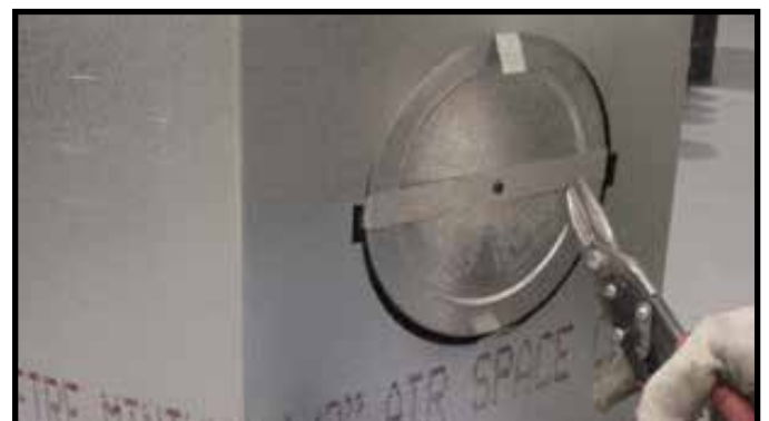
Figure 9.13 Cut the metal retaining band and fold the sides out.
