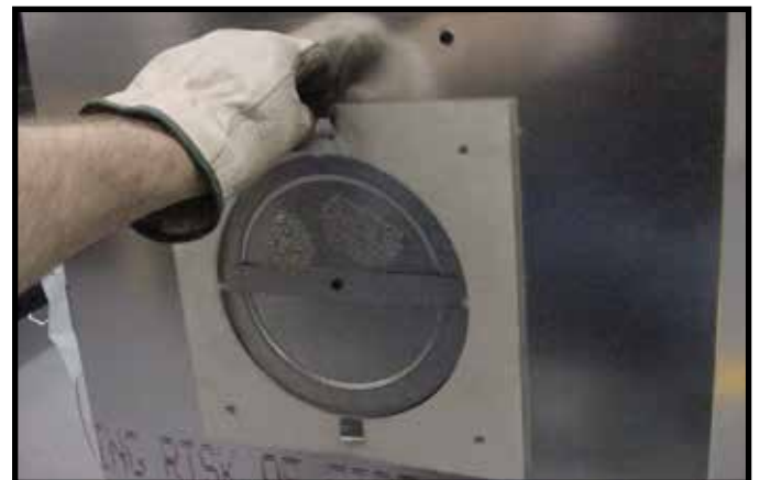
Figure 9.12 Fold the tabs toward the center of the fire plug (90°) and remove the insulation gasket.
