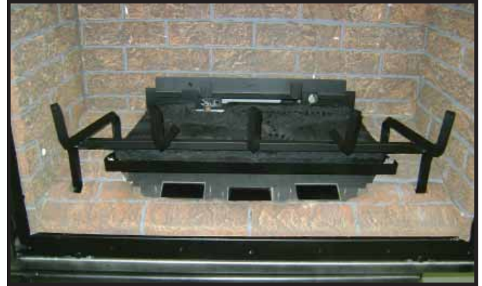
Figure 6. Front Base Refractory Installed
