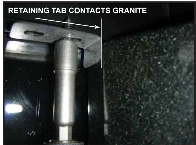
Figure 21. Placing Outer Corner Granite Trim Piece.
