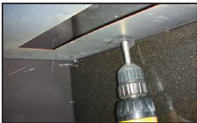
Figure 12. Fastening Angle Tabs to Secure Granite in Place.
