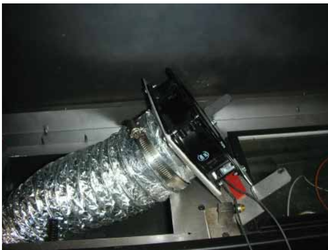
Figure 8.16 Blower Removal Through Hole in Firebox
