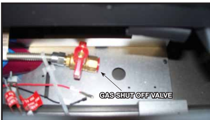
Figure 9.4 Gas Fitting Access
