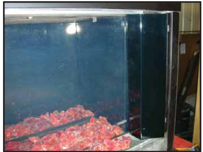
Figure 11. Installing Outside Corner Trim Piece onto Clip.
