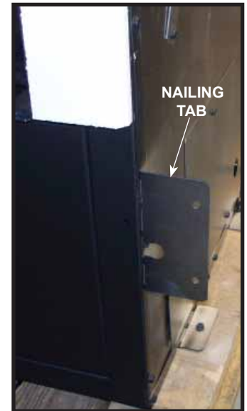
Figure 6.4 Nailing Tabs Installation Position
