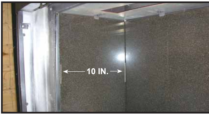
Figure 8. View of Back and Side Piece Installed.
