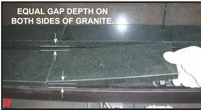
Figure 16. Installing Inner Front Granite Pieces.
