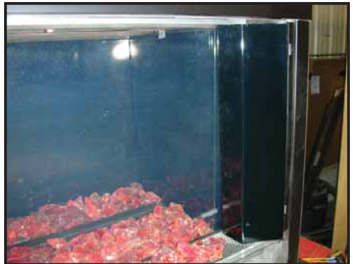
Figure 10. Outside Corner Trim Piece Installed.
