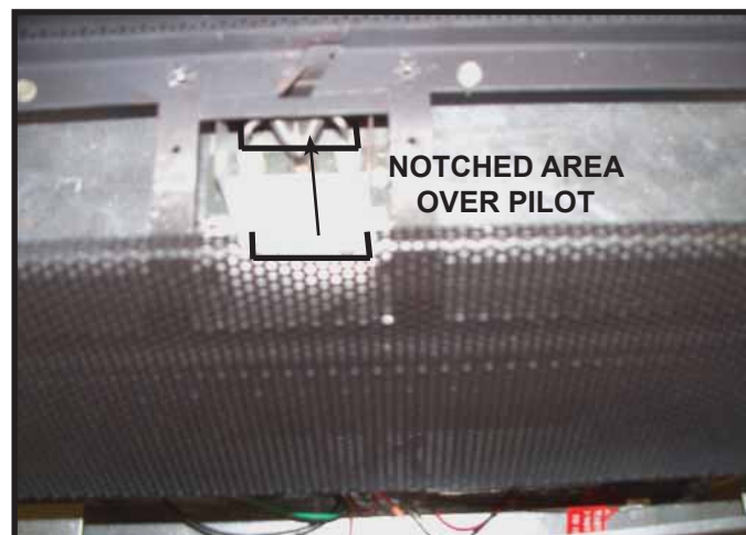
Figure 14. Installing Front Base Mesh Granite Support.
