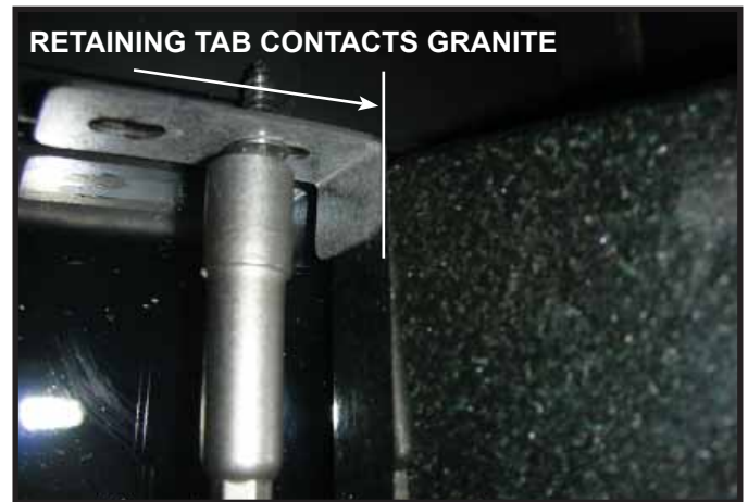
Figure 10. Placing Outer Corner Granite Trim Piece.
