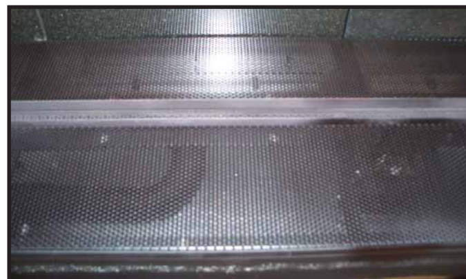
Figure 15. Base Mesh Installed.
