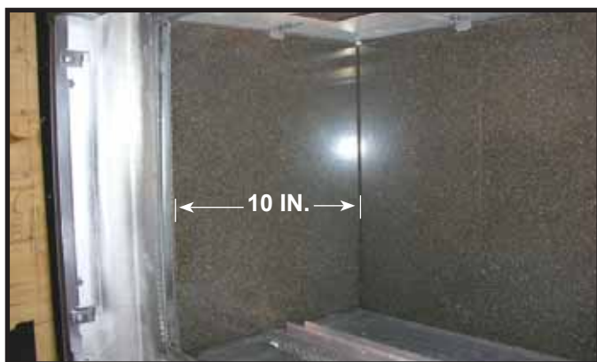
Figure 13. View of Back and Side Pieces Installed.
