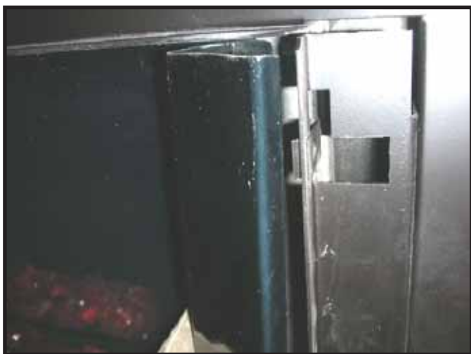
Figure 9. Installing Outside Corner Trim Piece onto Clip.
