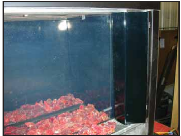
Figure 17. Outside Corner Trim Piece Installed.
