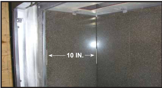
Figure 8. View of Back and Side Piece Installed.
