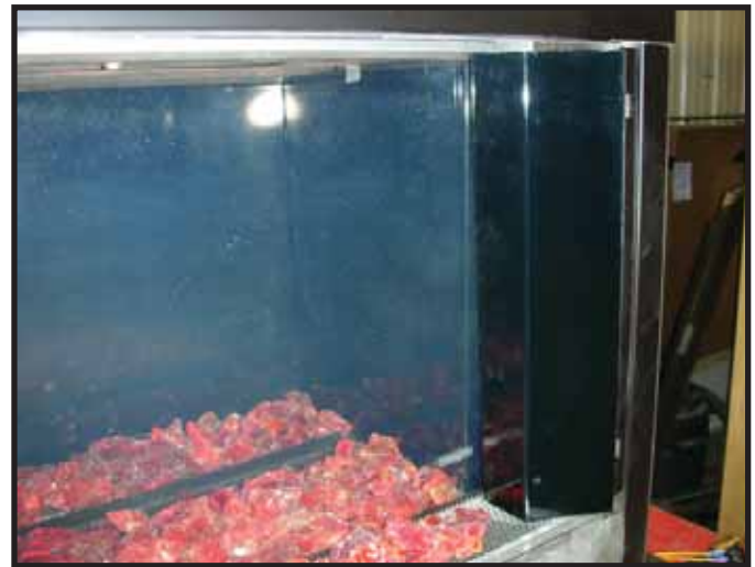
Figure 11. Installing Outside Corner Trim Piece onto Clip.
