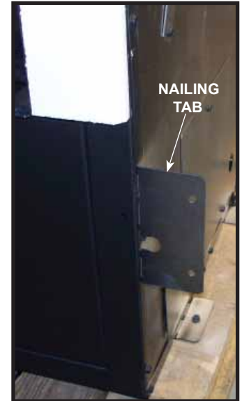
Figure 6.4 Nailing Tabs Installation Position
