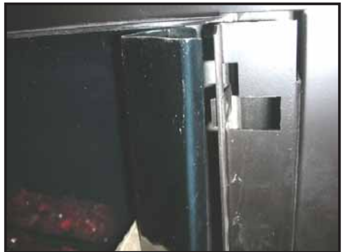
Figure 9. Installing Outside Corner Trim Piece onto Clip.
