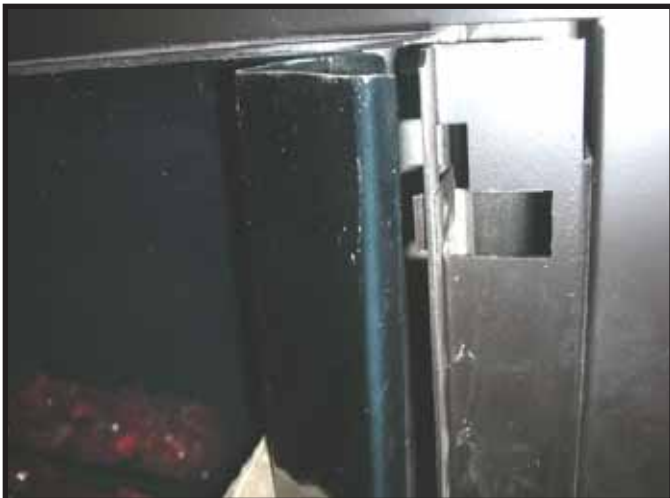
Figure 16. Installing Outside Corner Trim Piece onto Clip.
