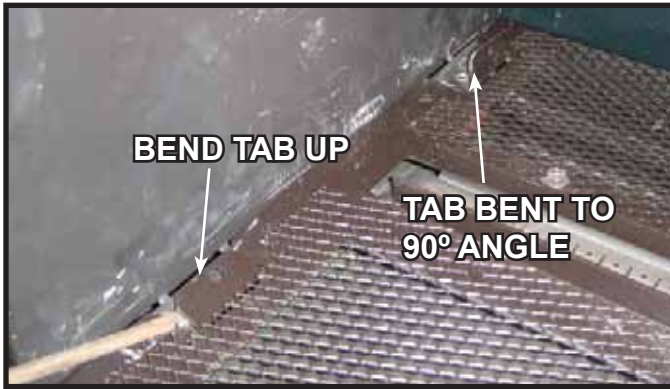
Figure 7. Bend Tabs Up to a 90 Degree Angle.
