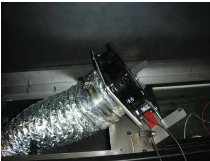
Figure 8.16 Blower Removal Through Hole in Firebox
