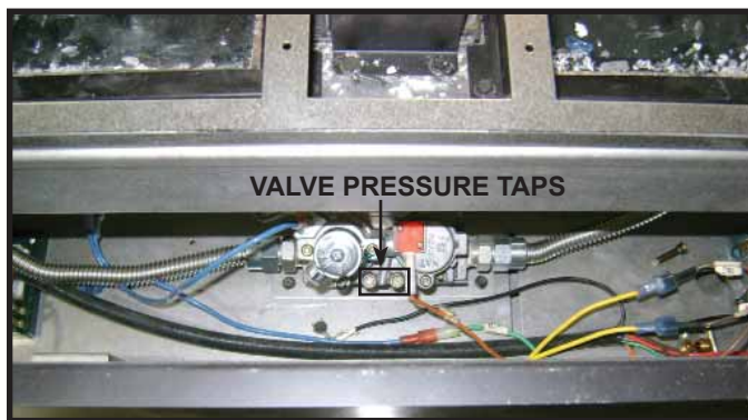
Figure 9.1. Valve Pressure Taps.
