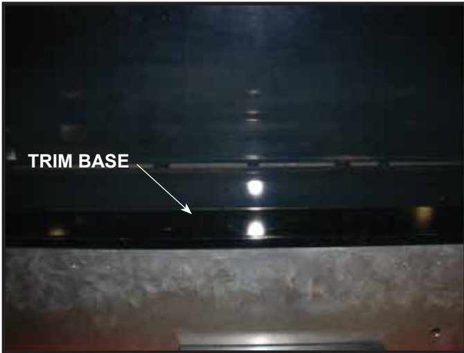
Figure 14. Porcelain Trim Base Installed.
