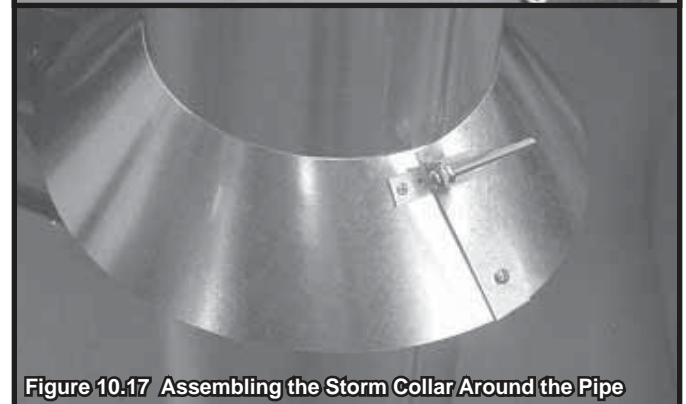
Figure 10.16 Assembling the Storm Collar
