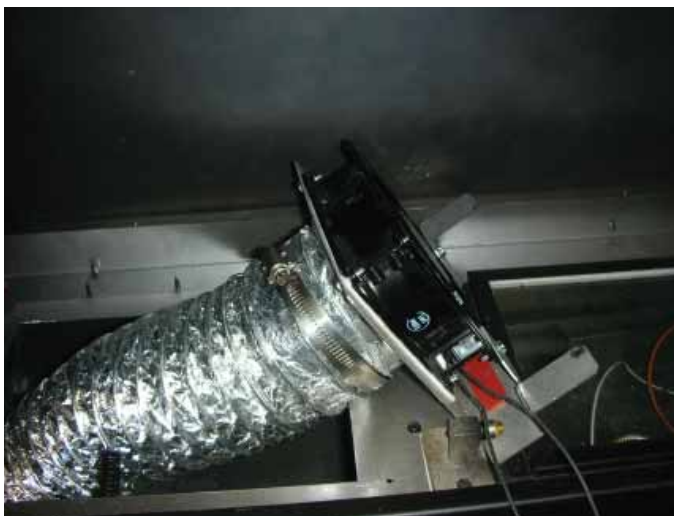
Figure 8.16 Blower Removal Through Hole in Firebox
