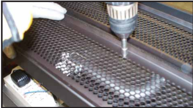
Figure 8.9 Removing Screws from Base Pan.
