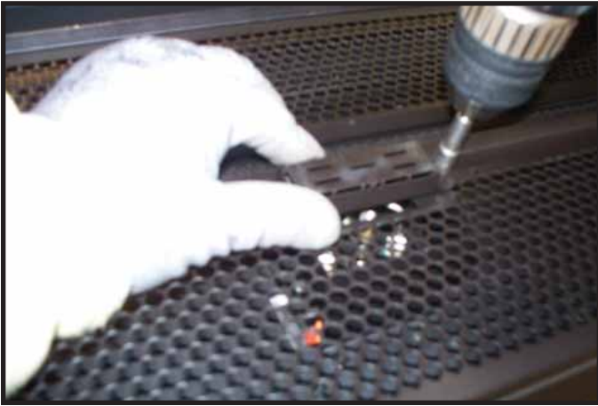
Figure 8.8 Removing Pilot Shield
