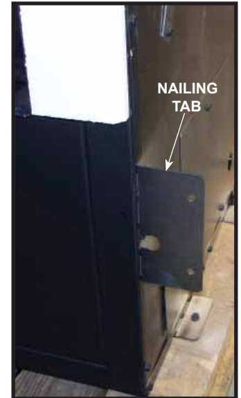
Figure 6.4 Nailing Tabs Installation Position
