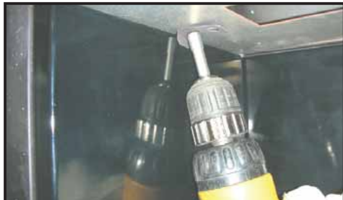
Figure 1.B.7. Installing Angle Tab to Secure Side Panel
