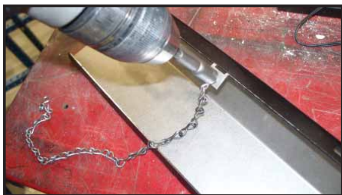
Figure 1.D.6. Attaching Chain
