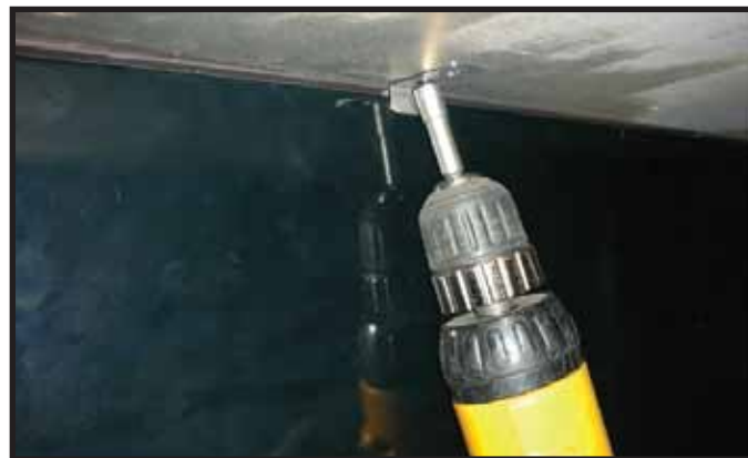
Figure 1.A.9. Fastening Angle Tab to Secure Back Panel
