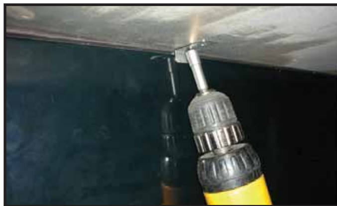
Figure 1.B.6. Installing Angle Tab to Secure Back Panel
