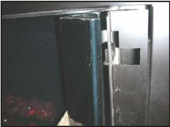
Figure 3.A.11. Installing Outside Corner Trim Panel onto Clip
