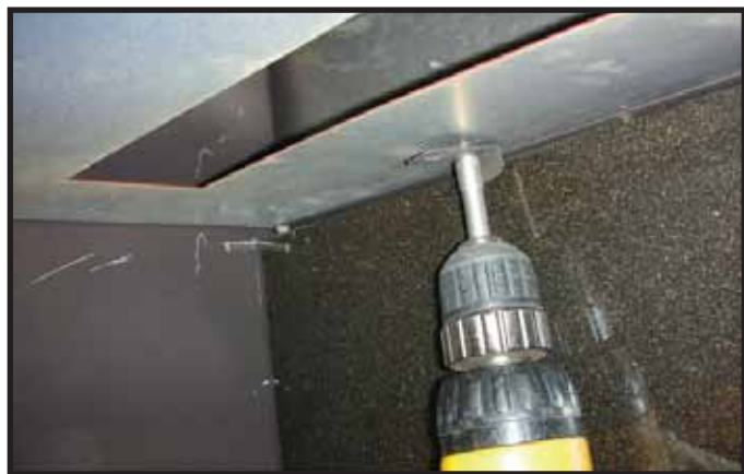
Figure 2.A.7. Fastening Angle Tabs to Secure Granite in Place
