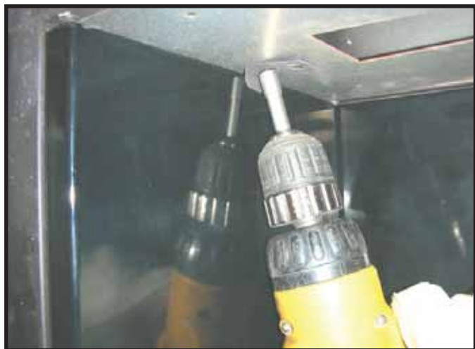
Figure 1.C.7. Fastening Side Panel with Angle Tab
