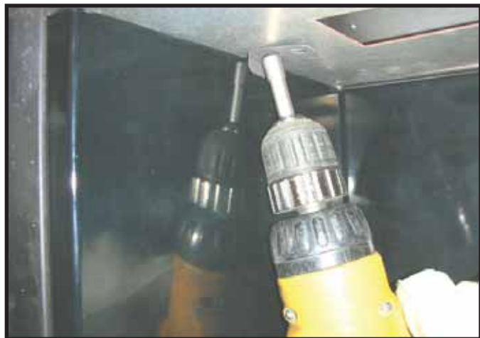
Figure 1.A.10. Fastening Angle Tab to Secure Side Panel
