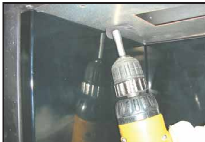
Figure 1.D.5. Fastening Side Panel with Angle Tab
