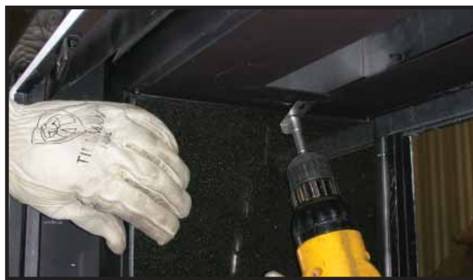
Figure 2.B.5. Secure Granite Sides with Angle Tabs
