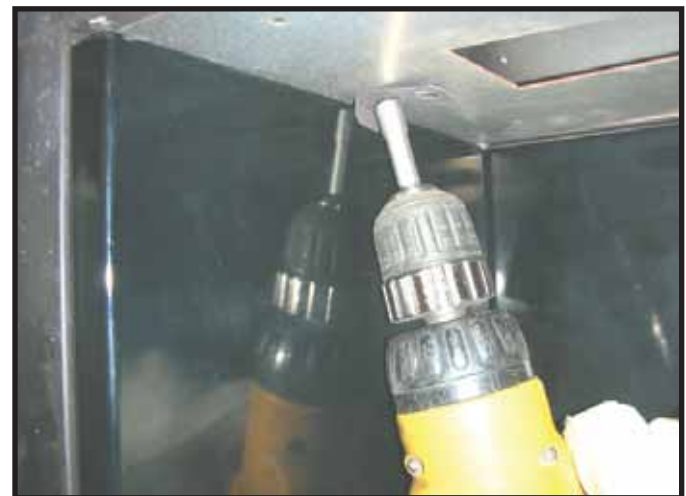
Figure 7. Fastening Side Panel with Angle Tab.
