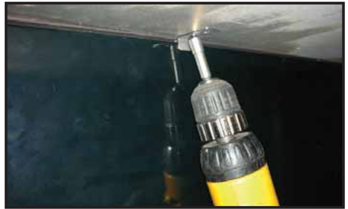
Figure 9. Fastening Angle Tab to Secure Back Panel.
