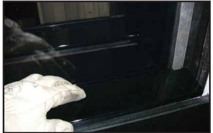
Figure 11. Install Outer Bottom Panel.
