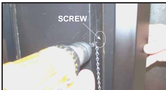
Figure 16. Attaching Chain.
