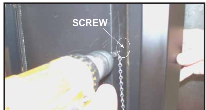
Figure 13. Attaching Chain.
