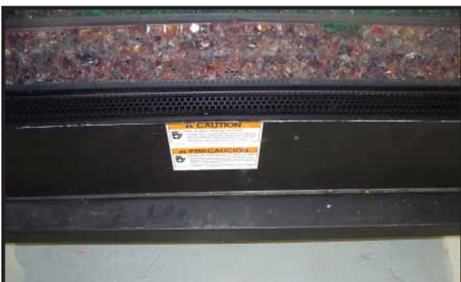
Figure 10. Access Panel Assembly Installed.
