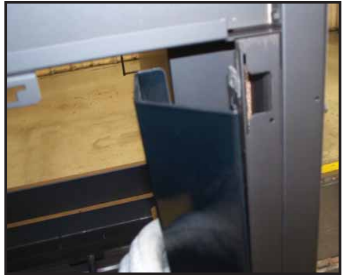
Figure 11. Installing Corner Panel onto Clip.
