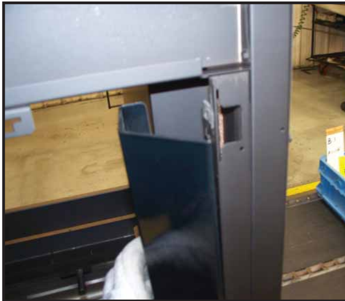
Figure 15. Installing Corner Panel onto Clip.
