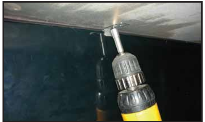
Figure 6. Installing Angle Tab to Secure Back Panel.
