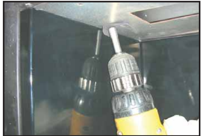
Figure 5. Fastening Side Panel with Angle Tab.
