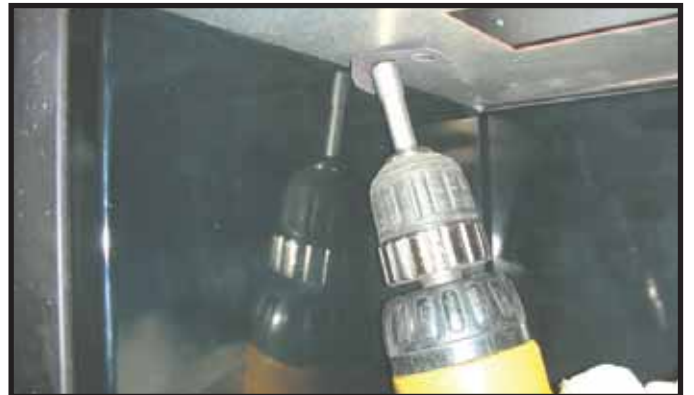
Figure 7. Installing Angle Tab to Secure Side Panel.
