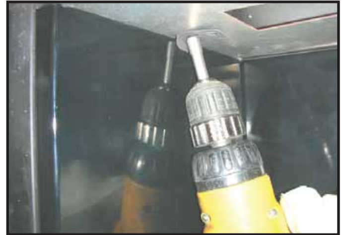
Figure 10. Fastening Angle Tab to Secure Side Panel.
