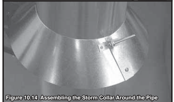
Figure 10.13 Assembling the Storm Collar
