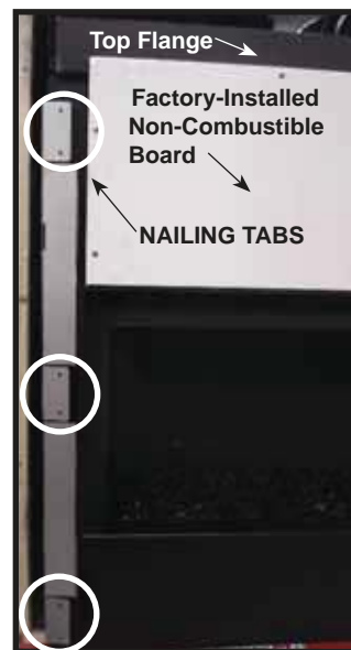
Figure 13.1 Nailing Tabs Shipping Position
