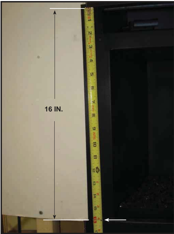
Figure 13.6 Confirm Fireplace Opening Dimension
