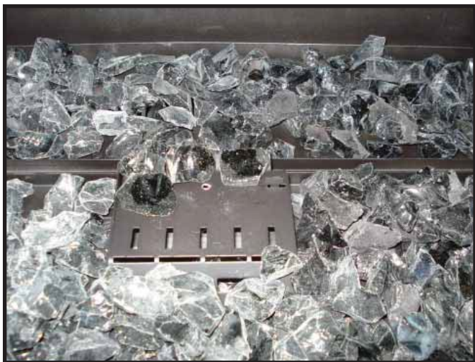
Figure 14.6. Place Flat Pieces of Rock Media
