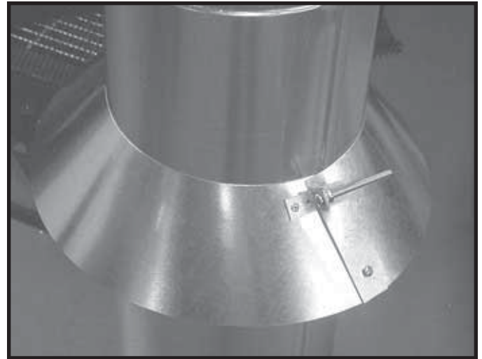
Figure 8.18 Assembling the Storm Collar Around the Pipe
