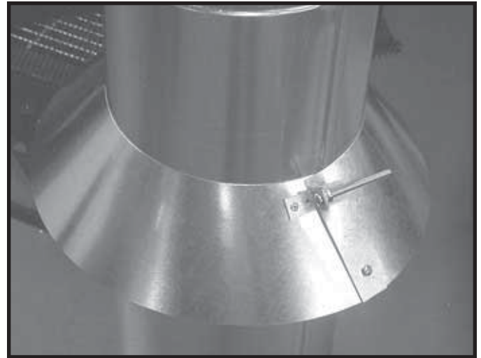
Figure 8.20 Assembling the Storm Collar Around the Pipe
