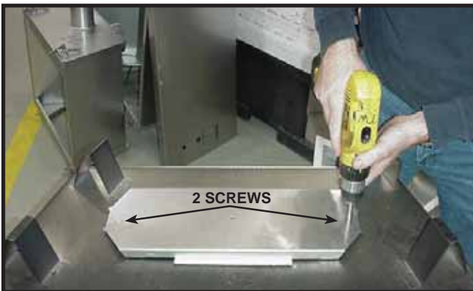
Figure 7.1 For top vent, remove the two screws holding the top heat shield in place. For rear vent, see Section 7B.
