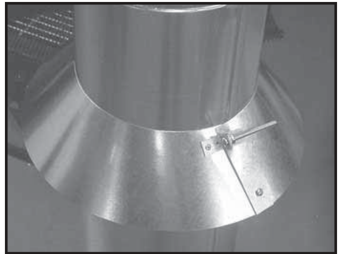
Figure 8.20 Assembling the Storm Collar Around the Pipe
