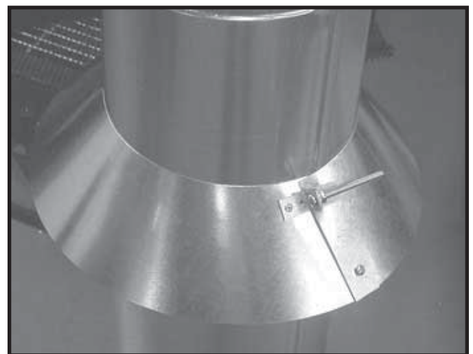
Figure 8.7 Assembling the Storm Collar Around the Pipe
